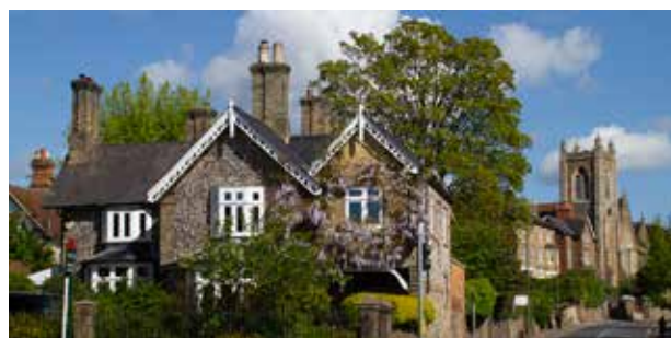
Architectural detailing: distinctive architecture and detailing
