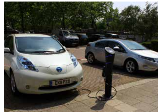
Electric car charging points
