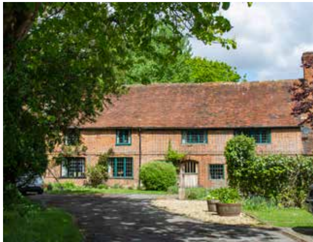
Old Manor Cottage, half of the original medieval Ash Manor House (Grade II* Listed), is located adjacent to the Ash and Tongham site
