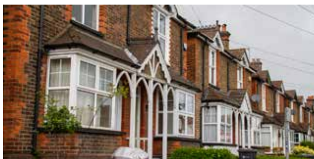
Architectural detailing: distinctive door detailing, bay windows, brick wall boundary treatment
